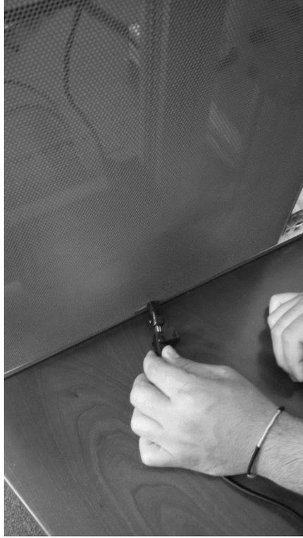
*Route the power cable coming from the actuator motor out the back of the unit through the notch in the back of the cover and attach the power cord extension.*
